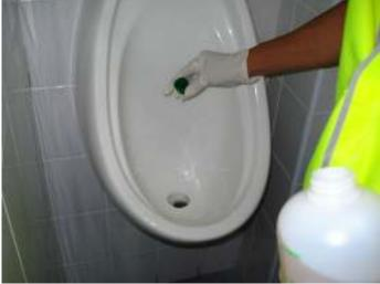
7. Put the plastic strainer at the bottom of the urinal
